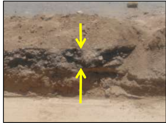
Photograph 4 Distribution of 0.7% Nano-modified emulsion through the sub-base layer
