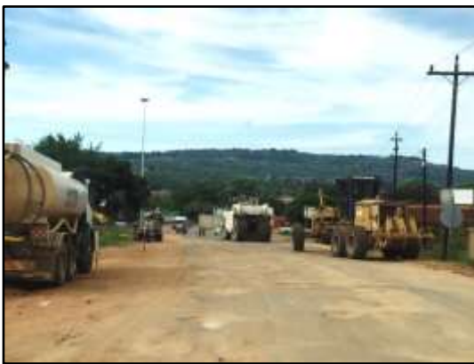
Photograph 5 Road condition with recycler in background, ready to start in-situ recycling
